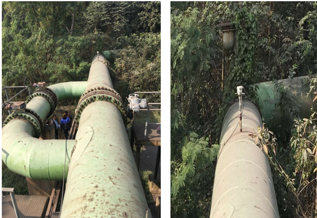
Figure 5.9 Flow meter installed at a location subjected to vibrations and insufficient upstream length
