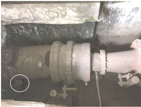
Figure 5.11 USFM installed at wrong location (without replacing the old venturi meter with a straight length pipe)
