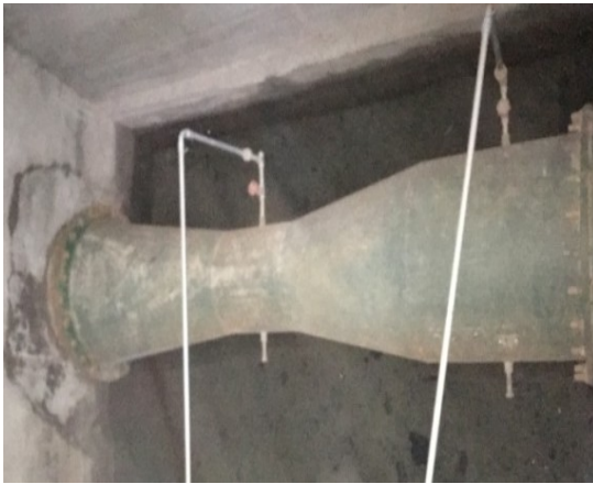
Figure 5.19 Venturi type DP flow meter
