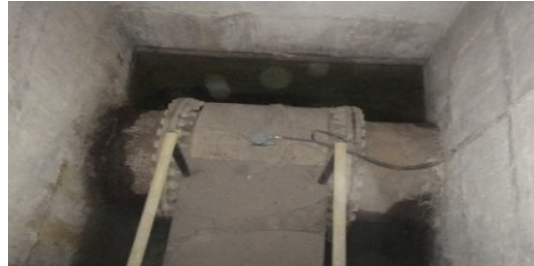
Figure 5.16 Electromagnetic Flowmeter installed at a flow measuring chamber
