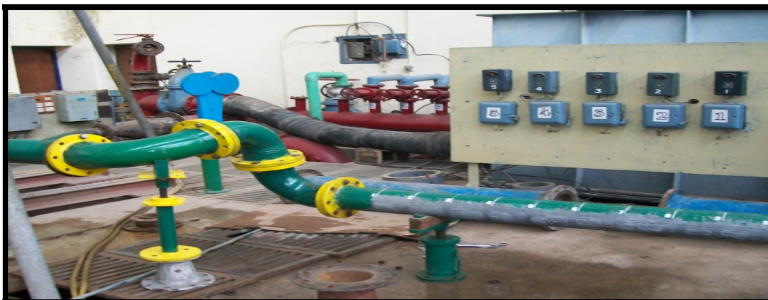
Figure 6.2: Upstream triple elbow out of plane
