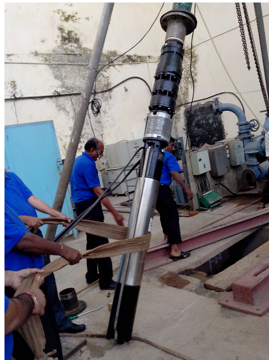
Figure 3.8: Submersible Pump Testing
