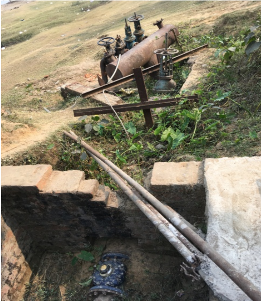
Figure 5.4 Water meter installed after series of flow elements
