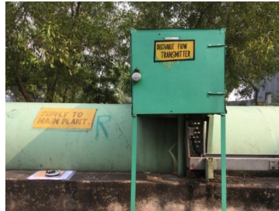
Figure 5.20 Pitot tube DP transmitter
