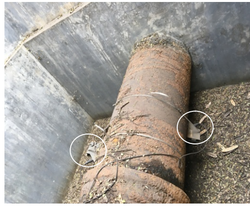
Figure 5.12 Poorly maintained clamp on type USFM (also no periodic calibration done)
