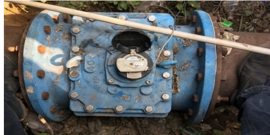
Figure 5.5 Water meter installed after reducer
