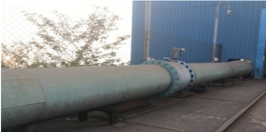
Figure 5.15 Electromagnetic Flowmeter installed at delivery line
